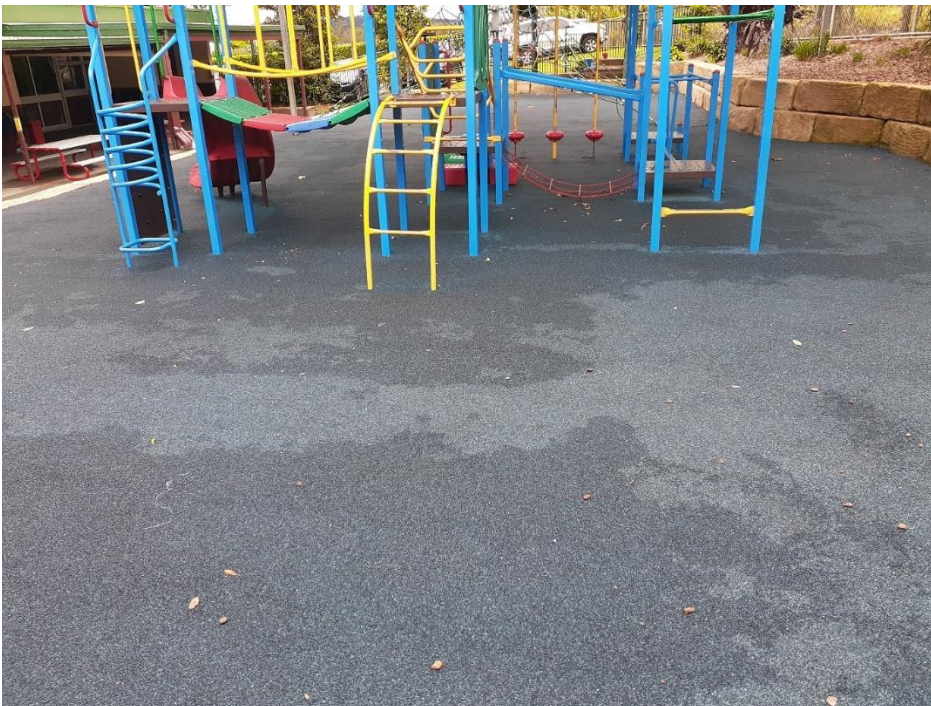
Photo 2 This area has a professionally placed synthetic soft fall ground surface in accordance with Australian Standards set out in AS/NZS 4422: and AS 4685.1.
