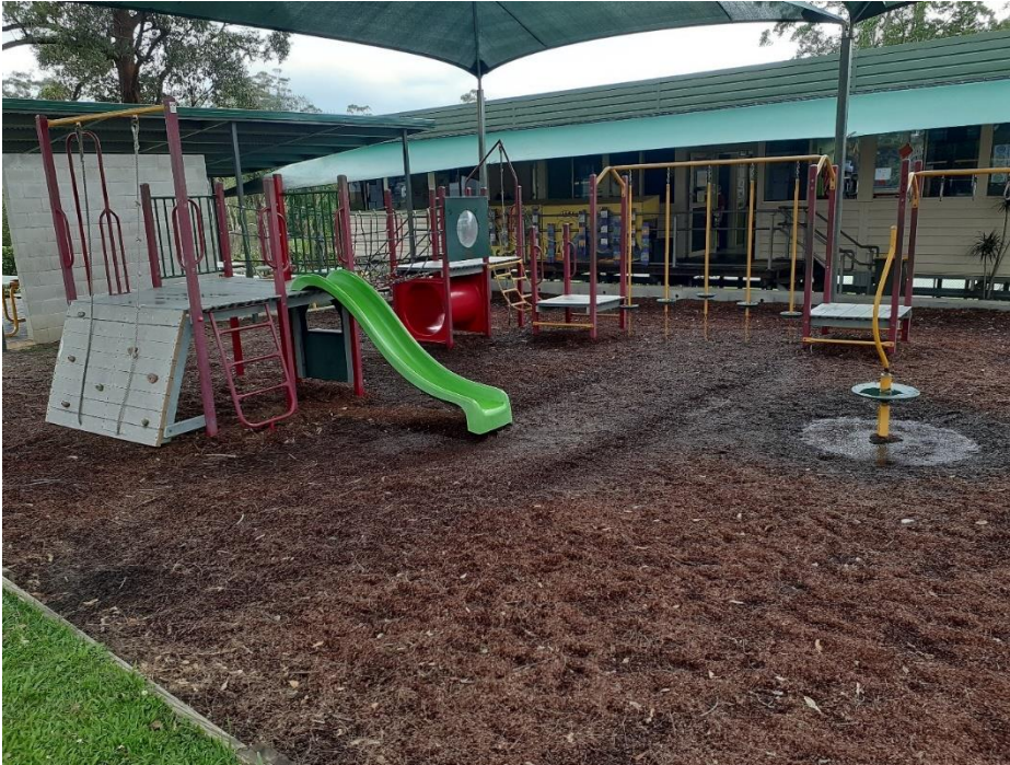
Photo 1 A playground area with bark soft fall. The soft fall material in this playground appears to be too thin to comply with current requirements. If a child were to fall from the playground equipment a possible broken bone or head injury could occur.
